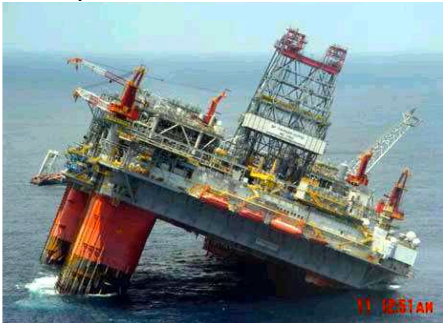
Figure 10: Thunder Horse platform tilted after Hurricane Dennis in 2005
